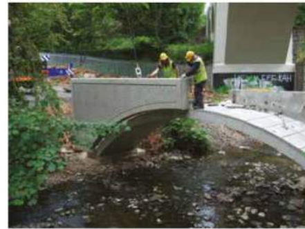
Figure 3.4 Use of pre-cast concrete segments for a bridge as a low-cost alternative to a culvert (courtesy WDR & RT Taggart)
